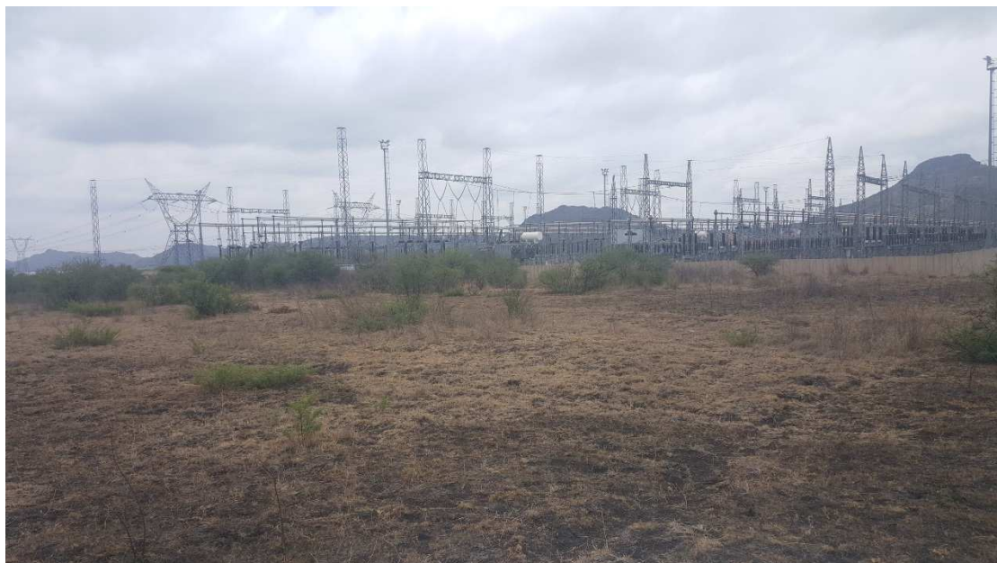
Figure 2-2 View across site to existing substation
