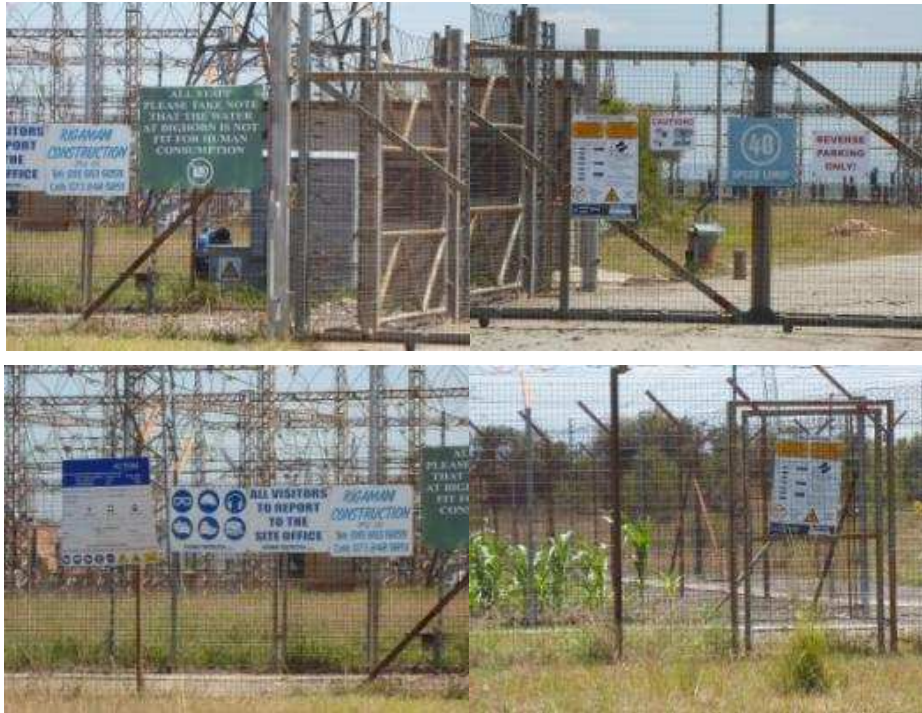
Figure 6-3 Health and Safety Warnings displayed on the perimeter of a substation
